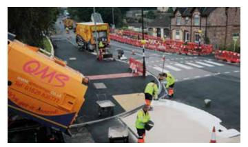
Following the completion of the civil engineering works, QMS mobilised to site and proceeded to install the line marking using a combination of Thermoplastic Screed and Preformed Thermoplastic Road Marking materials. These markings were installed by our trained and qualified workforce who carry an NVQ level 2 or 3 together with SSSTS or SMSTS qualification for site safety.
