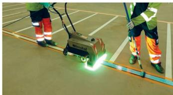
QMS was contracted to deliver over 8,000 metres of internal pallet line and safety walkway markings within a new distribution warehouse at Eurocentral near Glasgow in Scotland.
