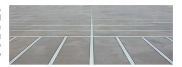
QMS RapidShield is able to be installed to concrete surfaces in temperatures as low as -28°C, so it can be installed within a working freezer environment. The finished product is impervious to most known substances including acid, oil and blood. With the system boasting solvent and VOC free attributes, it is possible to install markings within live food warehouses with minimal disruption to the client.
