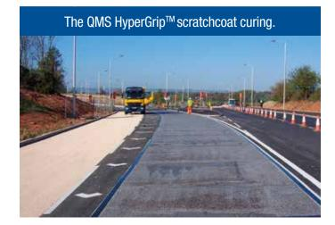
The QMS HyperGrip™ system for the contract required a scratchcoat void filler to be installed prior to the installation of the surface course. This was to ensure that the surface voids within the new bituminous substrates did not compromise the aesthetic appearance and functionality of the finished system. The scratchcoat void filler material is applied to the surface via a flat bladed squeegee and allowed to cure.
