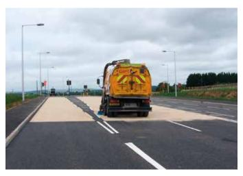
Following the completion of the QMS HyperGrip™ system, all Road Markings within the site constraints were replaced in accordance with BSEN 1436:2007 to the retro-reflectivity requirements of R2 (100mcd/m2/lux) and the skid-resistance requirements of S3 (SRT 55). This ensured minimum disruption to the road user and provided the client with a completed project without the need to return to site on many occasions with different resources.
